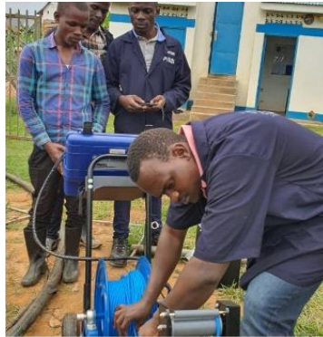
Inspection and regeneration of boreholes by the static plant team
