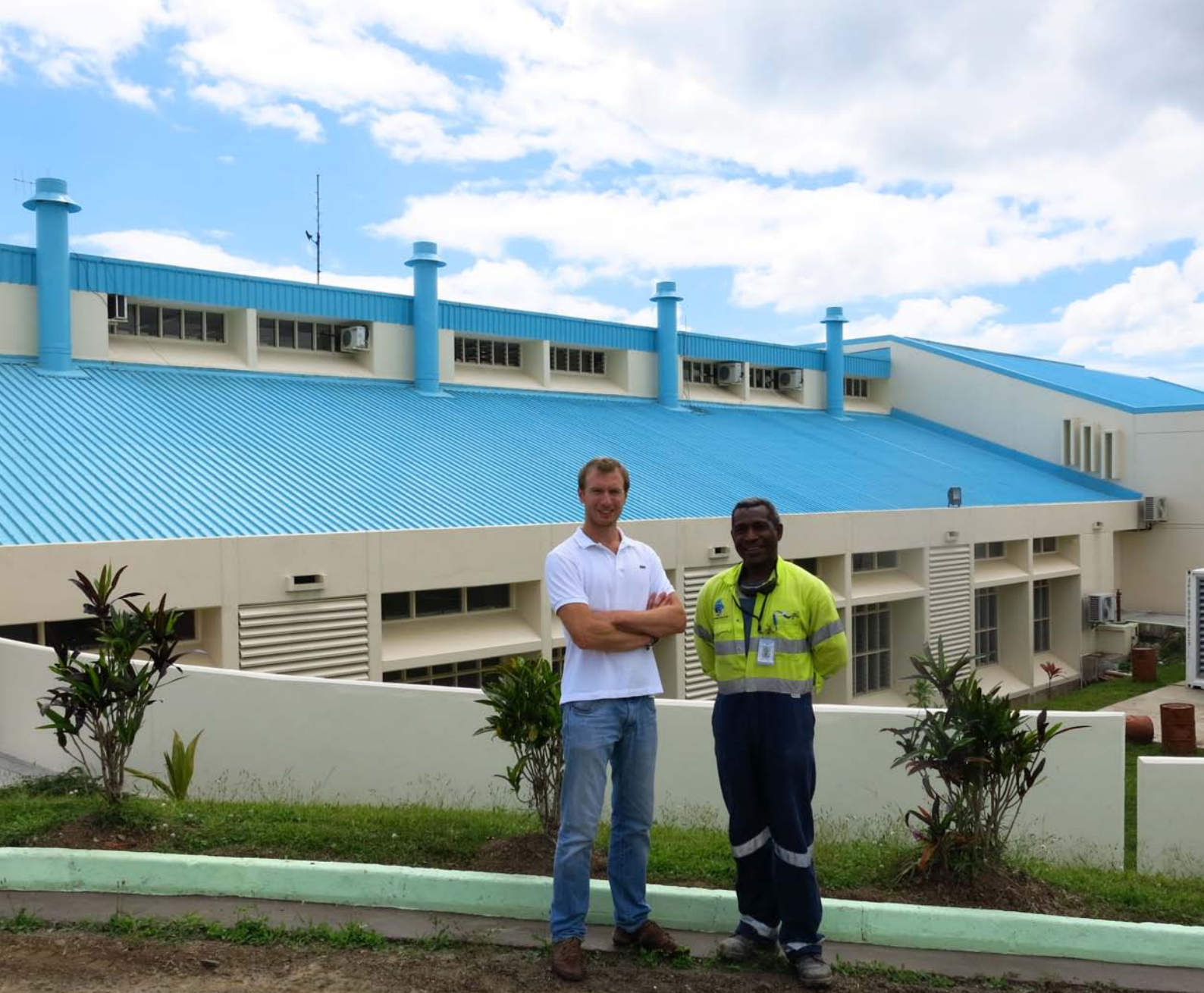
GWOPA Consultant (left) and employee of WAF (right) at Waila Water Treatment Plant
