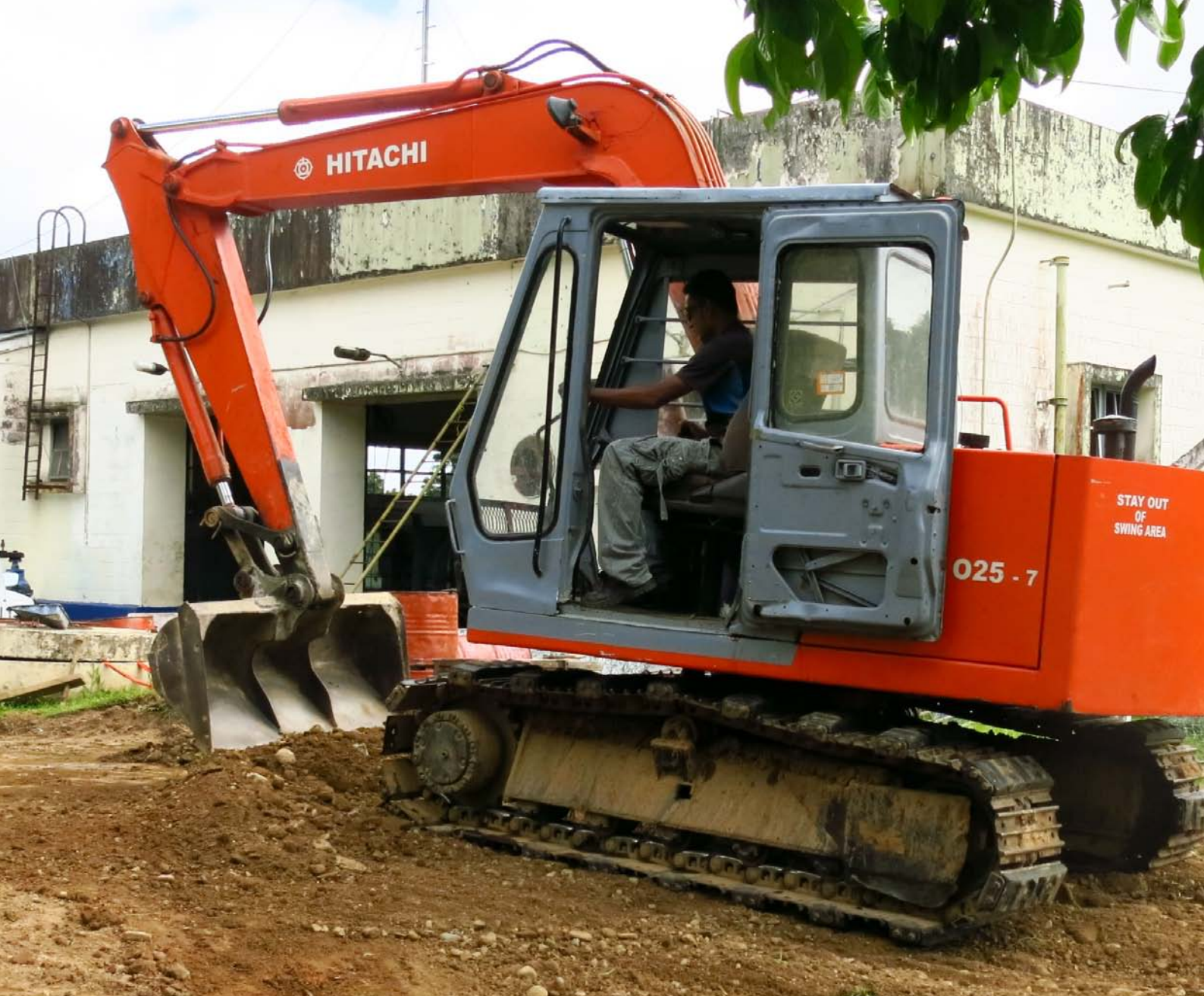
Levelling works at Waimanu water intake, Fiji Islands
